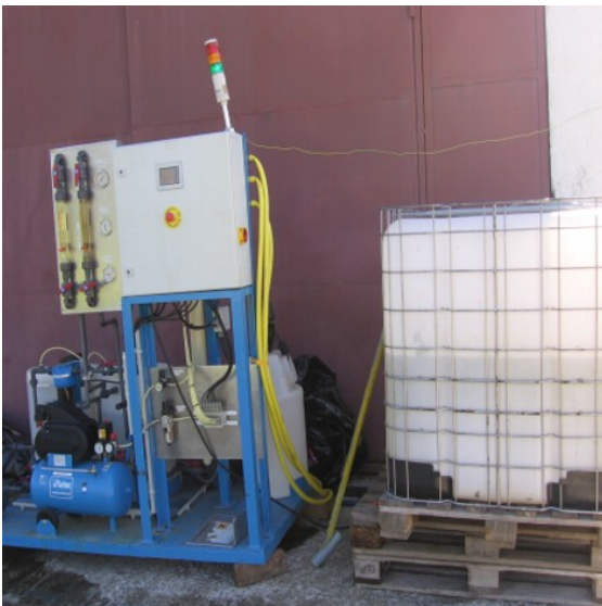
Fig.2. The image of microfiltration-ultrafiltration pilot plant
