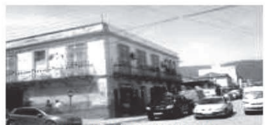
Photograph n°4. Colonial individual habitat (CIH)
