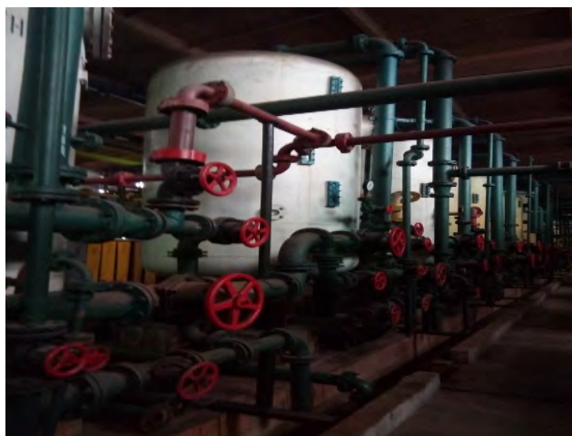
Fig. 3. View with ion-exchange filters
