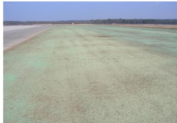
**Fig. 4.** The final STRIP treated soil (in particular, the hydro-seeding finishing treatment)
