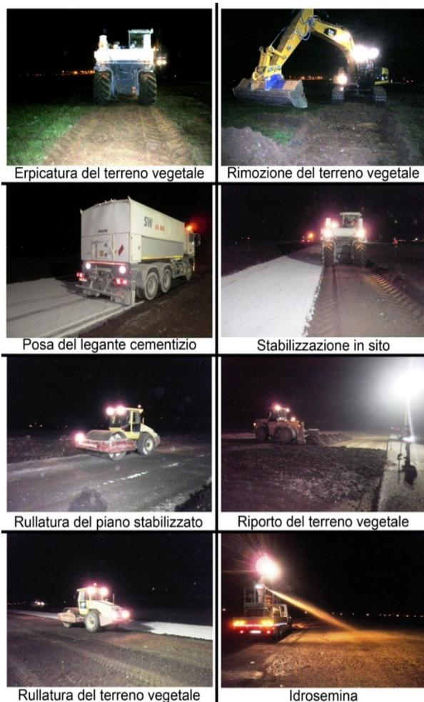
**Fig. 3.** Construction steps
