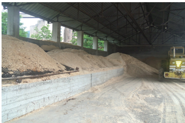
Fig. 6. The sawdust warehouse
