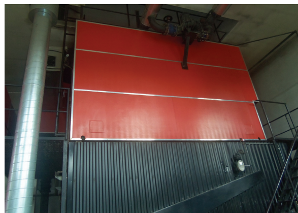
Fig. 7. The power plant tank
