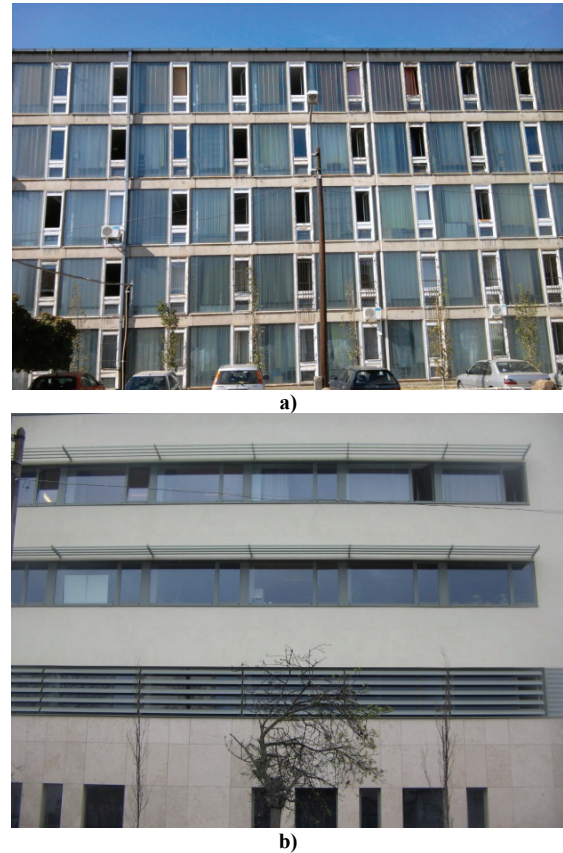
Fig. 6. East facade before and after refurbishment
